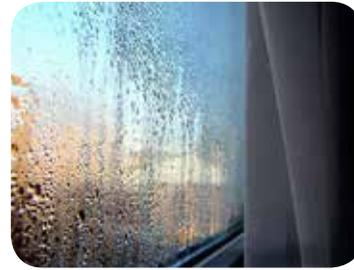
Black mould can't grow where salt deposits are present (as with rising damp) and is therefore a sign of condensation.
