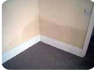
You can usually identify rising damp because it is often associated with a tide mark at the edge of the area of damp caused by salt deposits.
